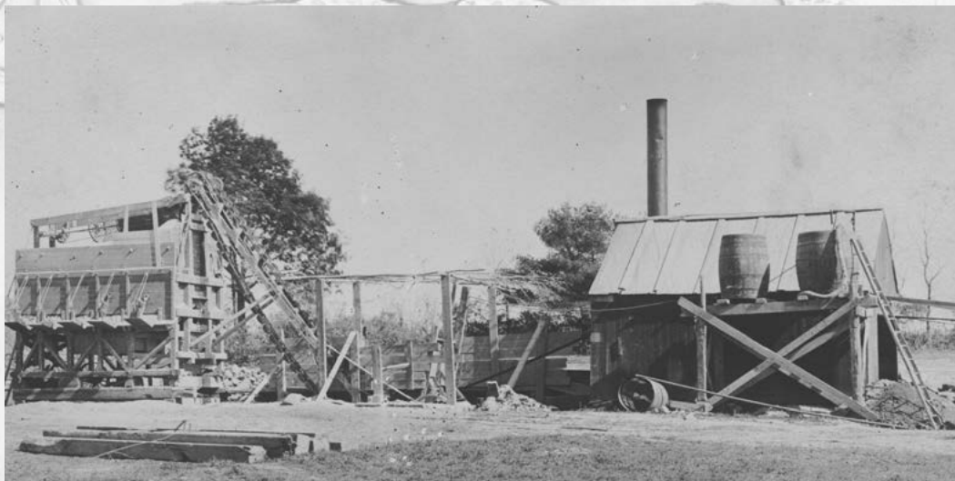
An important part of highway maintenance was the crushing of the stone. Stone crushers were set up as near as possible to the work sites to minimize the cost of material transportation which was done by horse teams.
