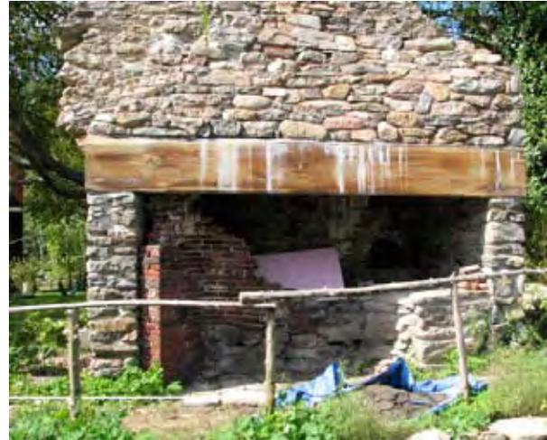
Figure 4.13: The current condition of the east side of the stone chimney with restored stonework and lintel and decaying later brick firebox, facing west.
