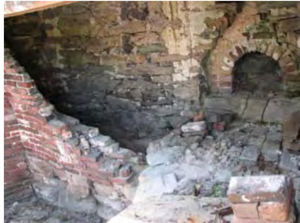
Figure 5.4: The opening for the original bake oven behind the later brick firebox insert in the east hearth.
