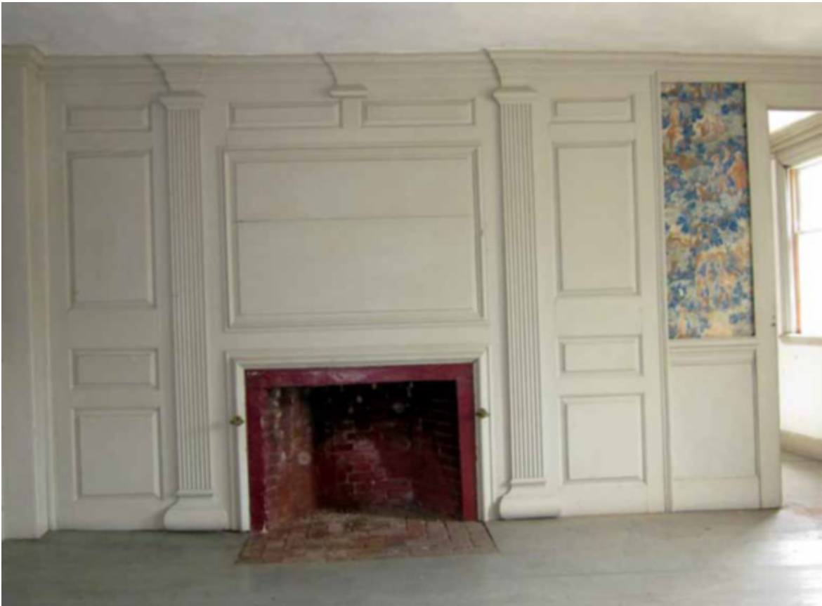
Four-panel doors replaced the flat board doors.
